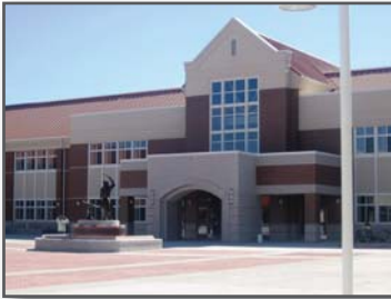
New Pittsburg High School Administration Building GC: S.J. Amoroso CM: RGM & Associates
